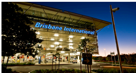
A series of PLS-900 are used at Brisbane airport, Australia
